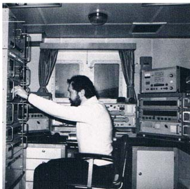
Funkraum der EXPLORA • Radio station of EXPLORA
